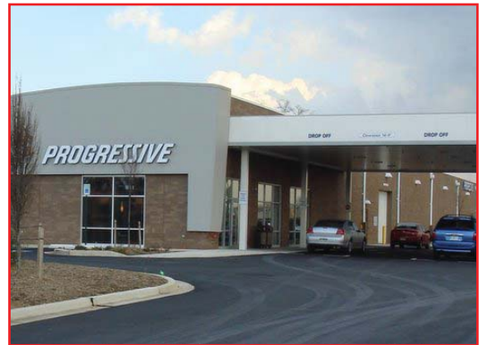
Progressive Claims Center completed
