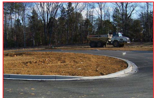
Edelen Village E&D completed
