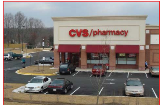
CVS at Highbridge completed
