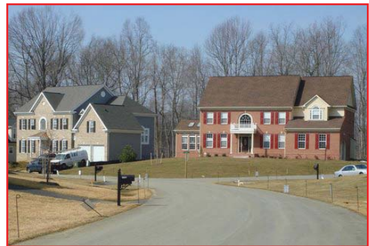
Oak Creek completed
